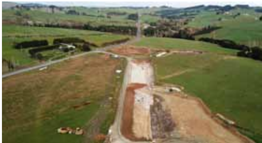
West end of site preparatory drainage and earthworks
